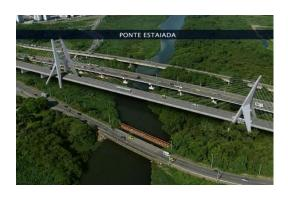
**Description:** As part of the Olympic Project in Rio de Janeiro, the Ayrton Senna Stayed Bridge was designed and built by 2013-14. Terratek was in charge of the site investigation, foundation design, quality control through integrity and pile loading tests. All foundations were piled with 2.5 to 3 m diameter bored piles socketed in rock.
