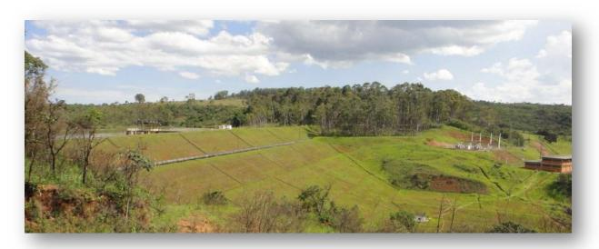
**Description:** Soledade Dam and its water reservoir is a large structure and part of the Gerdau Steel Manufacturing Plant. Soledade Dam was built in the 70s and is a large 70 m high compacted earth dam. Terratek is in charge of the dam safety analyses and since 2006.
