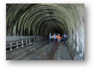
**Description:** Existing tunnel, built by 2011 with concrete lining spalling, excavated through hard rocks, 40 m<sup>2</sup> cross-sectional area, 3 km long. The purpose of the tunnel is to accommodate gas pipelines.
