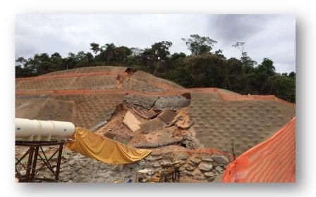
**Description:** Road tunnel, 120 m<sup>2</sup> area, which failed in 2015 close to one portal.
