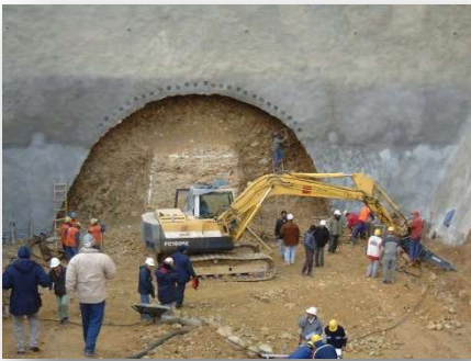
Cerrillos tunnel, Bolivia
