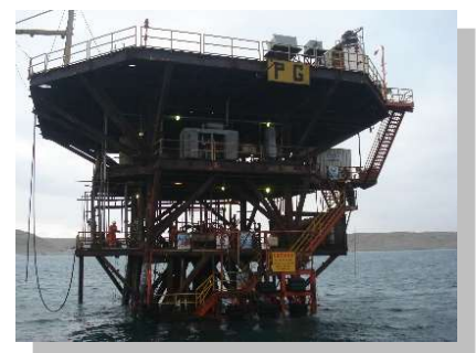
Offshore structure, Talara, Peru
