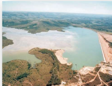
Morro do Ouro Tailings Dam
