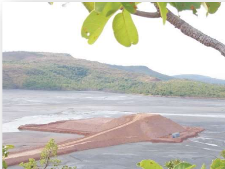
Trial Embankment on tailings
