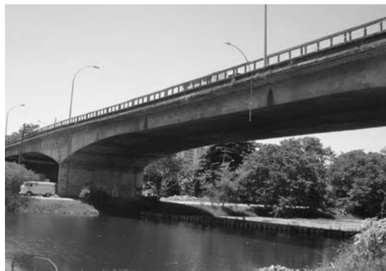
Figure 1: Bridge “Ponte do Canal de Sernambetiba”
