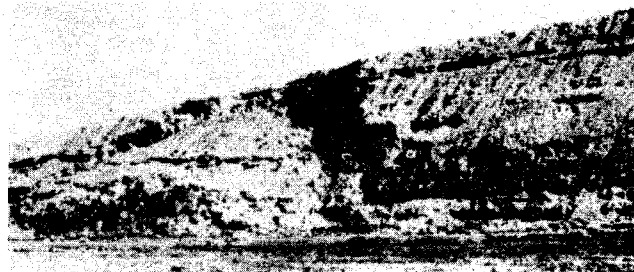
FIG. 1. Failure in OC Tertiary Clay Excavated Slope
